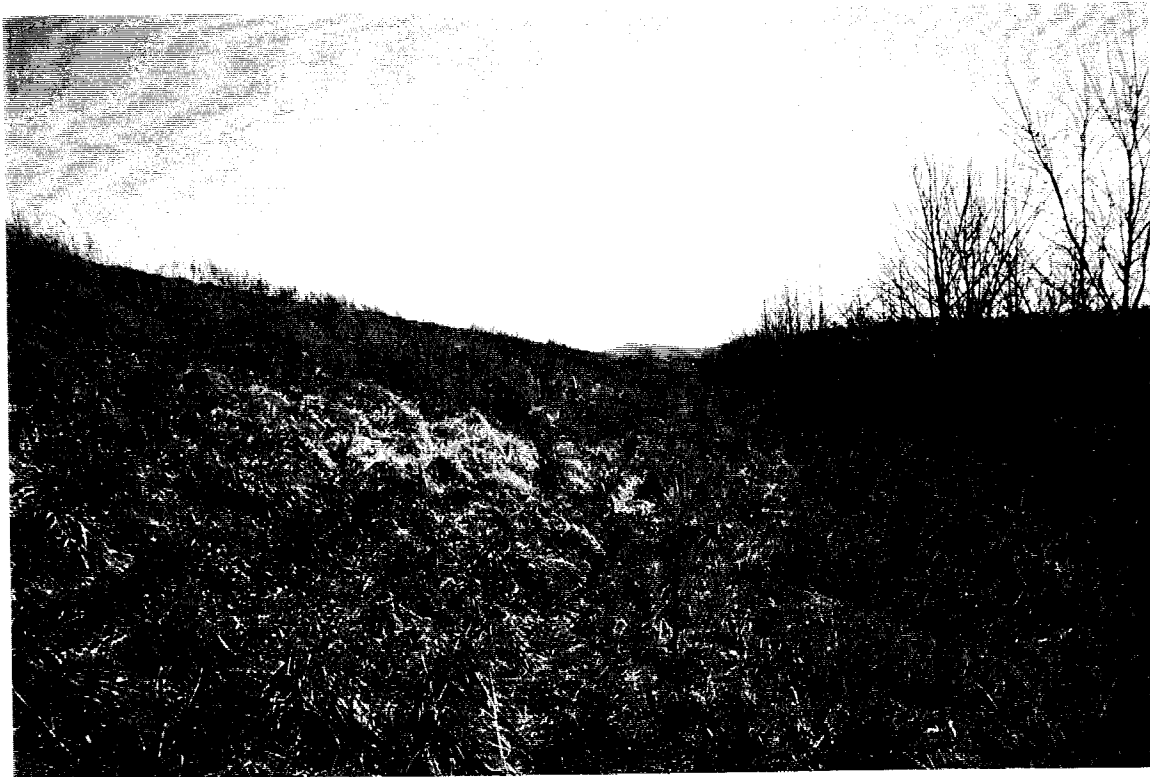
Figure 3. Southwestern dike in good condition with excellent vegetative cover.
