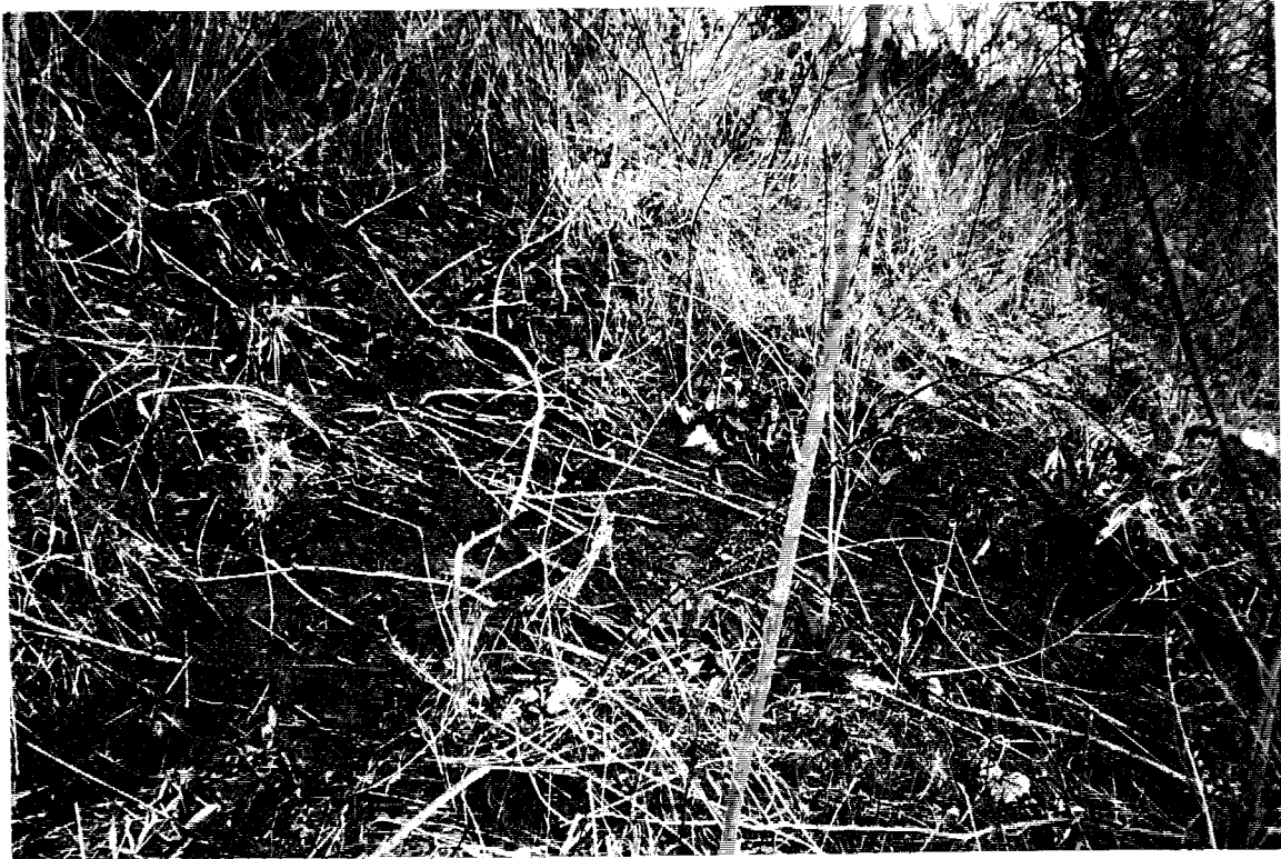
Figure 1. Seep area along eastern dike.
